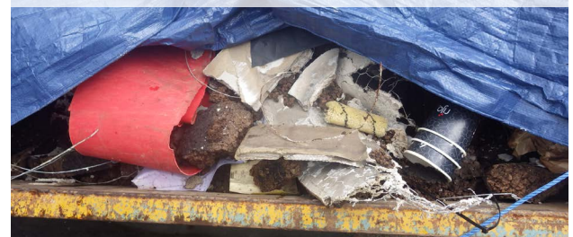
Top: The former plant room with asbestos debris on the pipes and floor. Bottom: Asbestos was left in an open skip.
