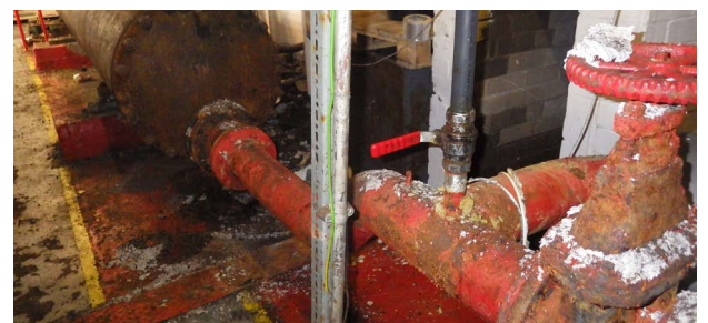
Top: The former plant room with asbestos debris on the pipes and floor. Bottom: Asbestos was left in an open skip.
